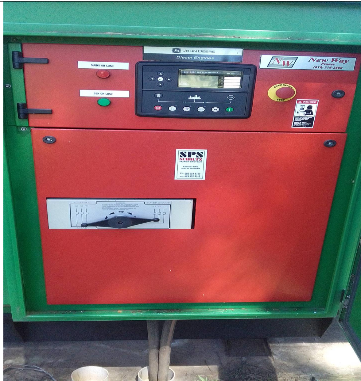
Figure 3: Control panel of the generator
