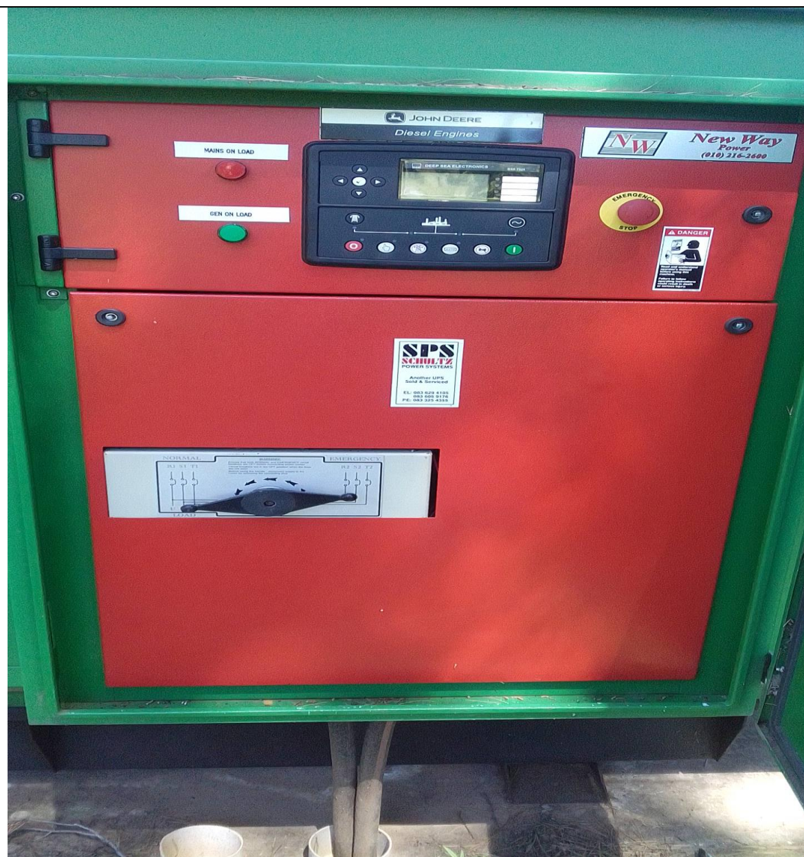
Figure 3: Control panel of the generator
